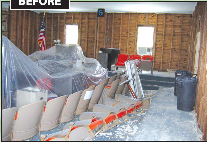
The lodge room stripped to the wall joists.
