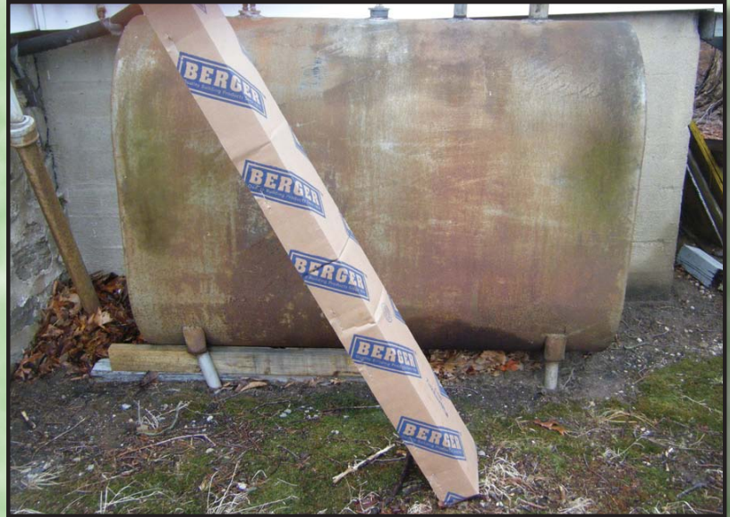
Replace oil with gas and add air conditioning.
